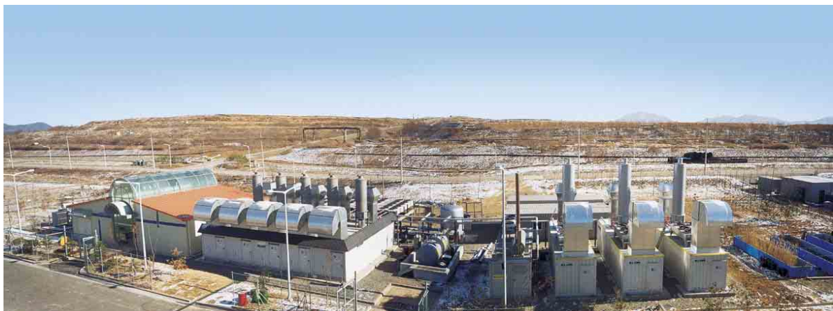
Fig. 1: Cogeneration plant with 9 containerized CHP modules on the Sudokwon landfill site (Korea)
