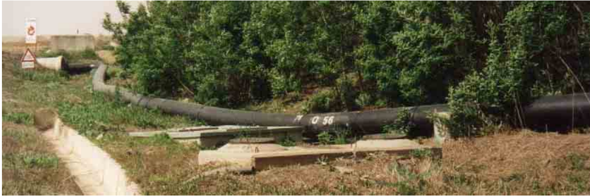
Fig. 2: Old circular pipeline, Area 1
